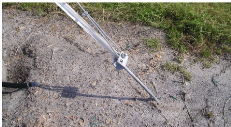
The ground anchors are the same types used to keep mobile homes secured.
